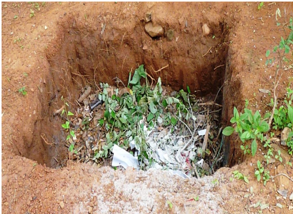
Waste Management Pit under Construction
